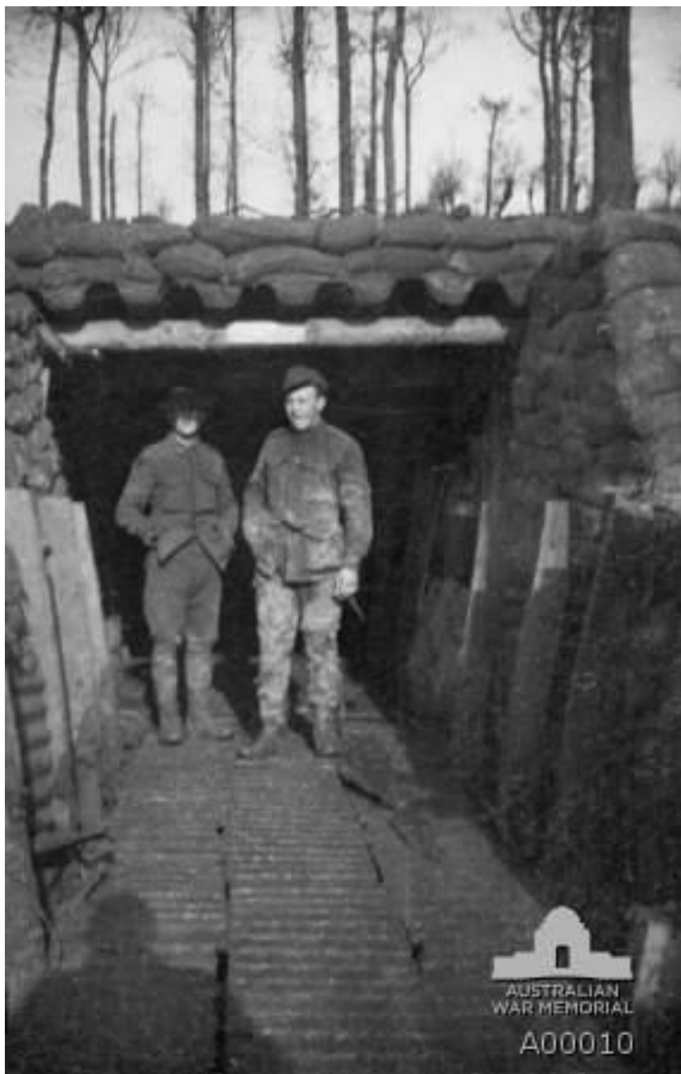
Two soldiers of the 23rd Battalion, 4144 Sergeant Edward Moodie and 1961 Albert Oswald Rix MM , standing at the entrance to the Catacombs, Hyde Park Corner, a system of tunnels of considerable length which were fitted to accommodate over 1,000 men. (January, 1918)
